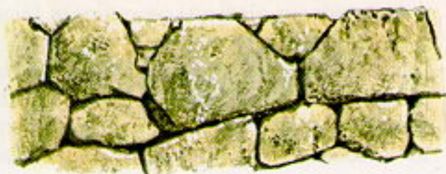
Above Etrusco-Roman arched gate, at Santa Maria di Falleri. Below Wall of polygonal masonry, Segni. When this masonry was used, gateways often had sloping sides and were either pointed at the top or had a long lintel across.
